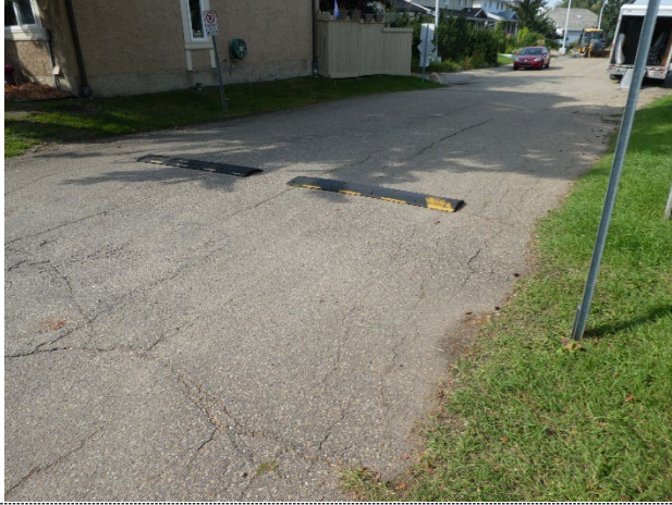
Asphalt roadway between north & south
