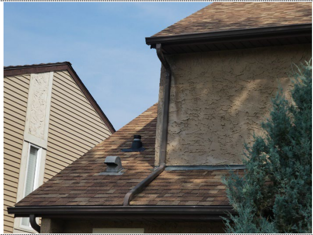
Upper downspout terminating into lower eavestrough
