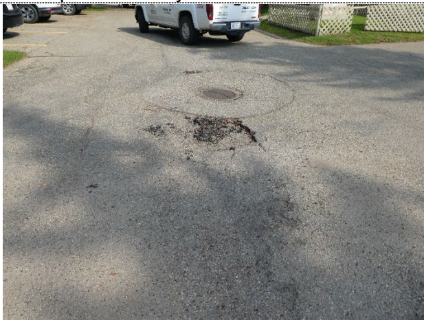
Deteriorated asphalt
