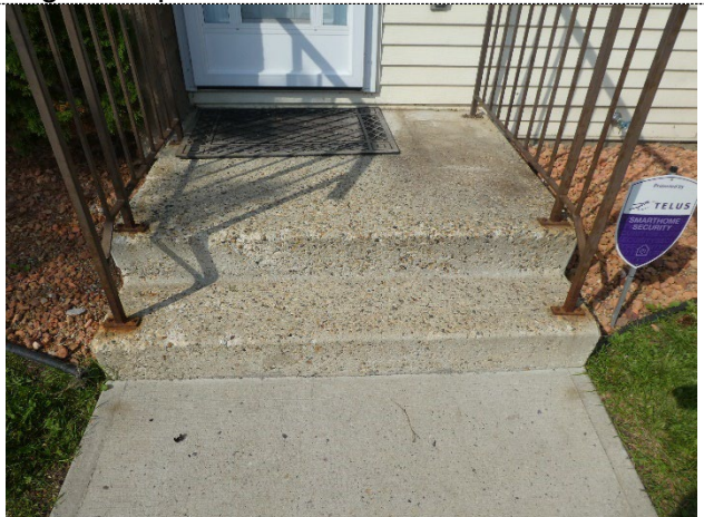
Significant spalling on steps
