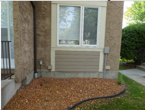
Wood siding & trim
