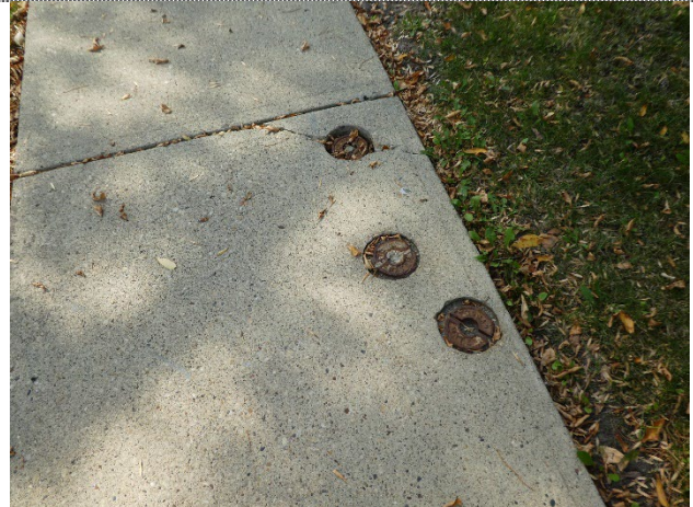
Shut off valves in walkway
