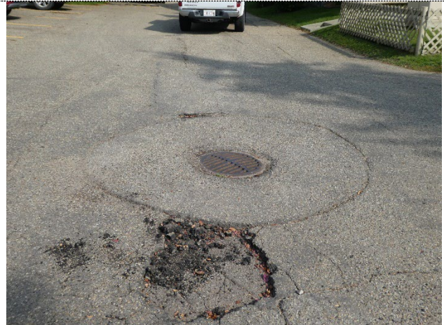
Drain in roadway
