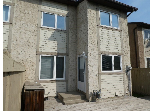
Back unit windows
