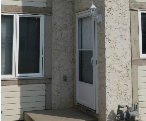
Typical back entrance door
