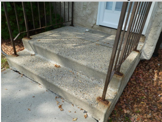
Significant spalling on steps
