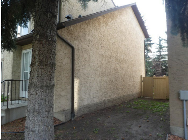
Stucco at end of building
