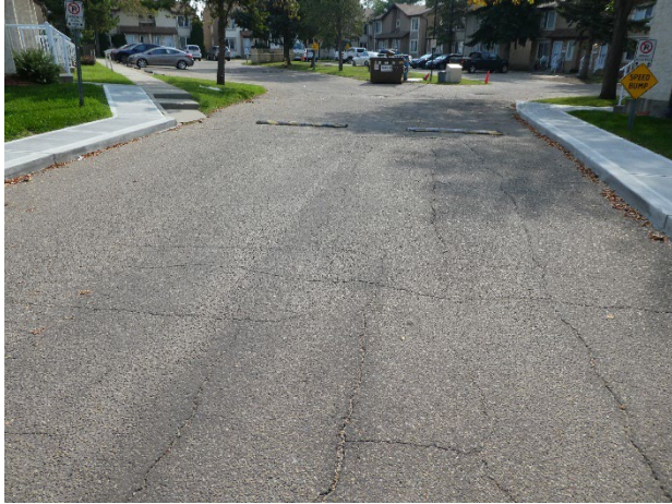
Asphalt roadway at entrance
