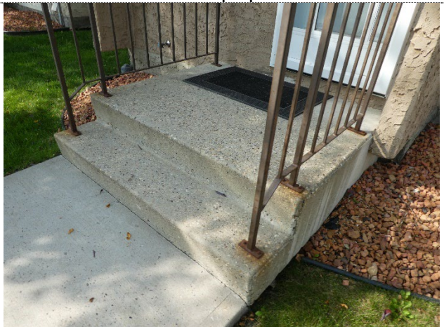
Significant spalling on steps
