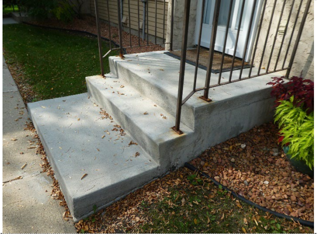
Replaced front steps
