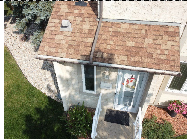
Shingle roofing
