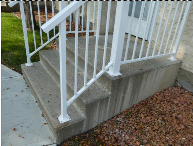
Front entrance step in fair condition – replaced railings
