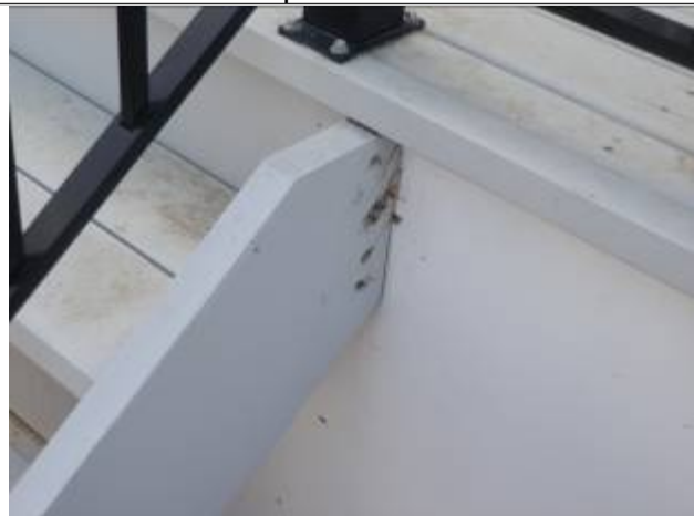
Minor deterioration at joints where screws penetrate
