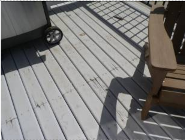
Deterioration at joints where screws penetrate
