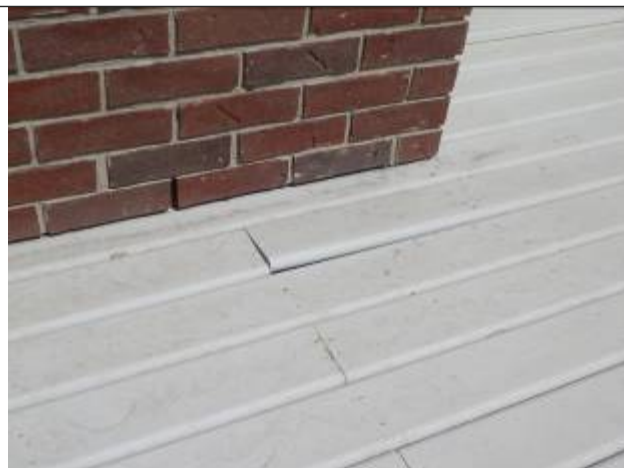
Deteriorated wood
