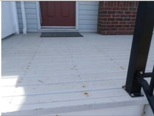
8 Rusted screws and bolts
