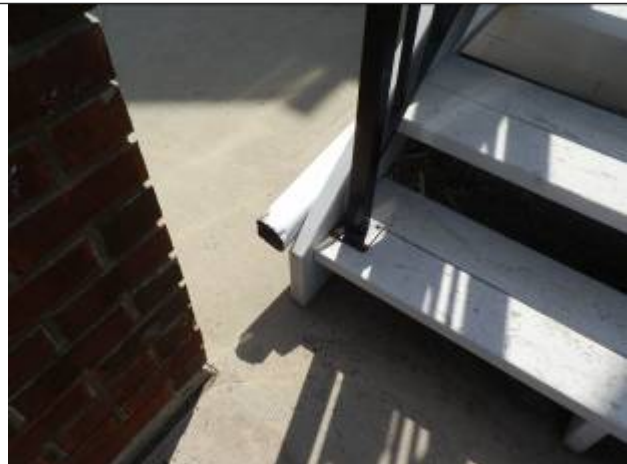
8 Downspout terminating against stringer
