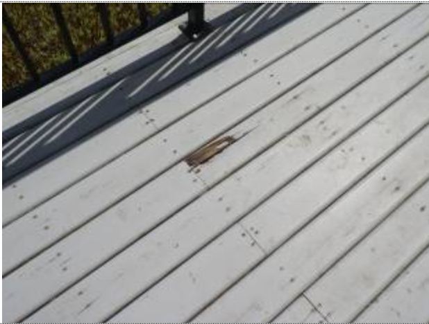
Deterioration at joints where screws penetrate
