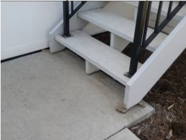
Deterioration at joints where screws penetrate
