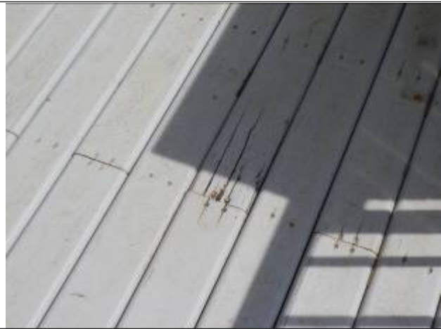
Deterioration at joints where screws penetrate
