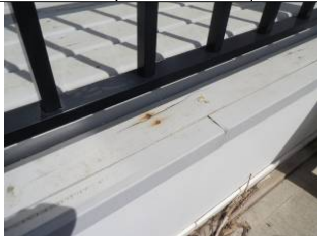
Deterioration at joints where screws penetrate
