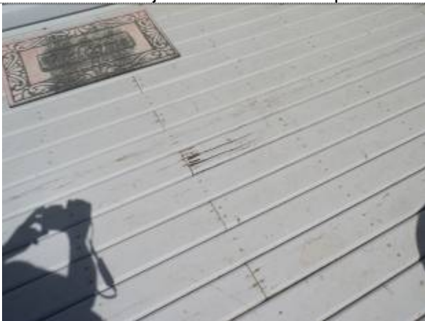
Deterioration at joints where screws penetrate
