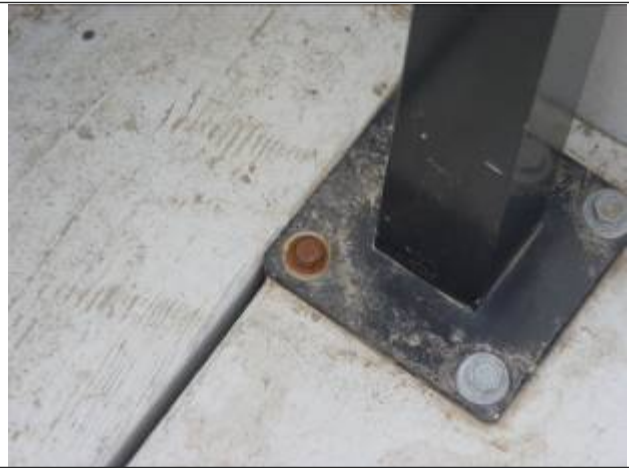
8 Rusted screws and bolts
