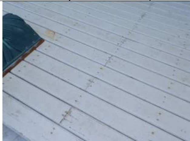
Deterioration at joints where screws penetrate
