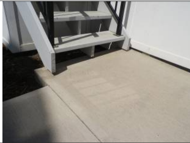
Steps do not rest on concrete
