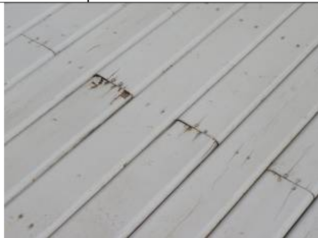
Deterioration at joints where screws penetrate
