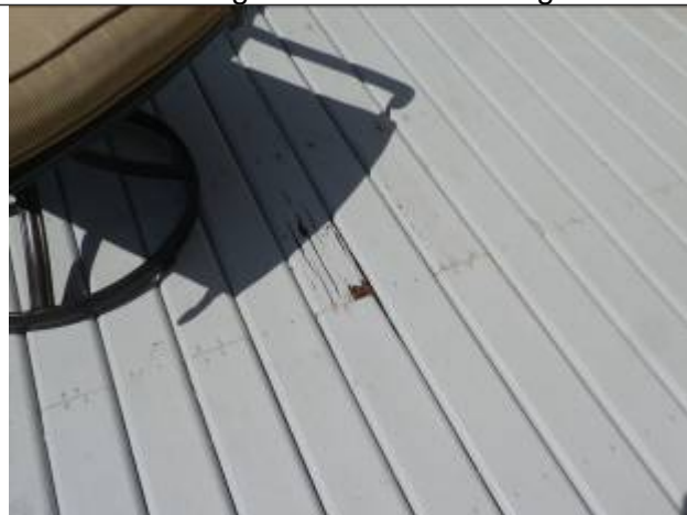
Deteriorated wood
