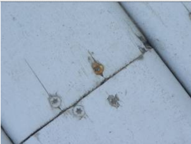
Only one screw rusting – suspect incorrect screws used
