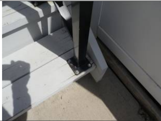
Damaged tread under railing
