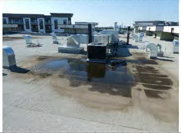
Significant ponding
