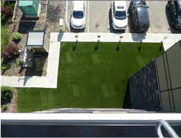
Parkade membrane below artificial grass on north courtyard area
