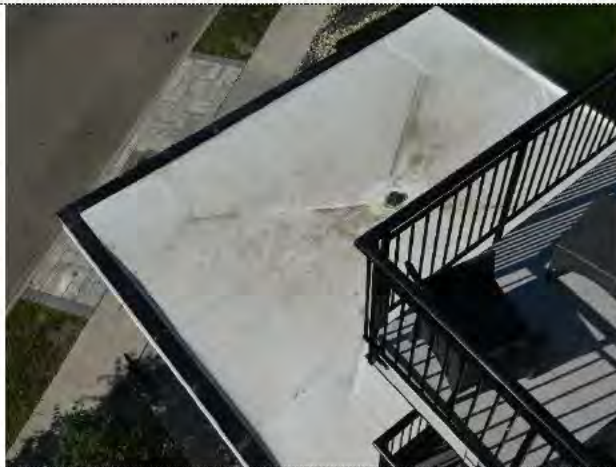
Front entrance canopy roof
