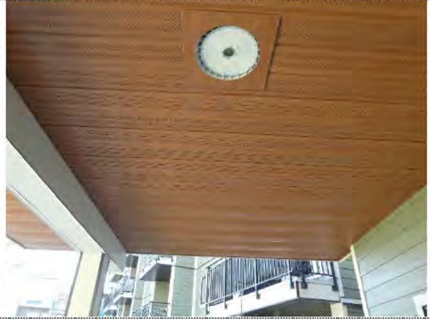
Soffit below canopy roof
