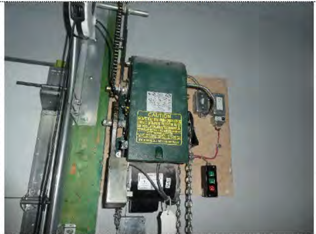
Garbage room overhead door & opener/motor
