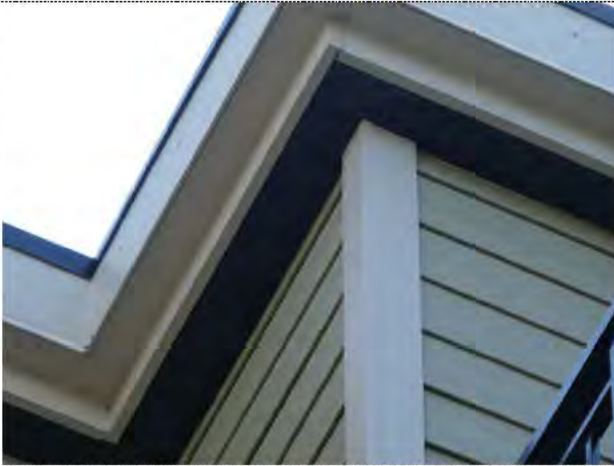
Soffit at roof perimeter
