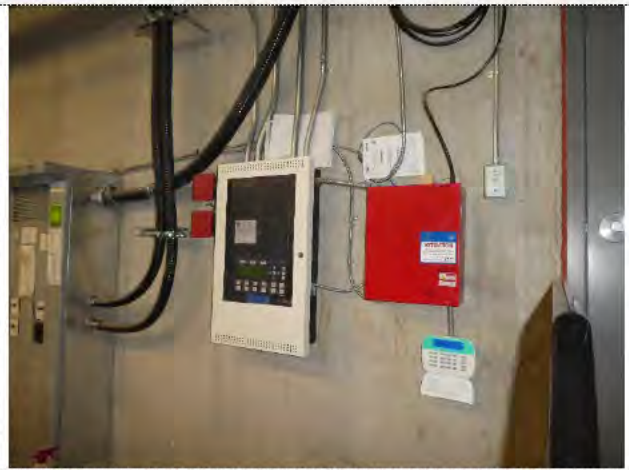
Fire alarm notifier panels
