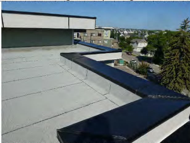
SBS roofing & cap flashing at parapet wall
