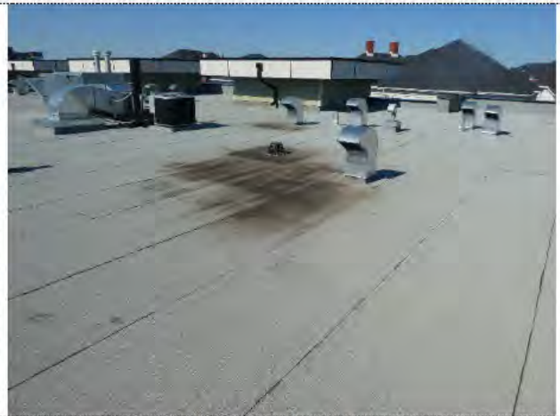
Main roof - SBS
