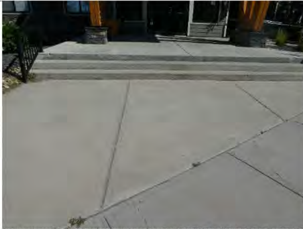
Front entrance walkway & steps
