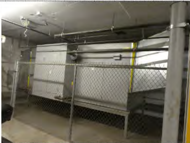
Engineered Air Parkade Makeup Air Unit M: HE451 S: S57515 MUA-1
