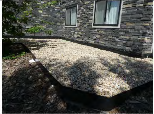
Parkade membrane below gravel SW front of property
