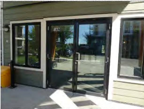
Front entrance doors
