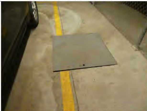
Sump pump location
