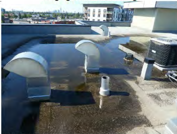
Significant ponding
