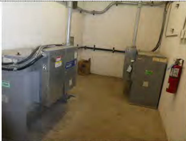
Elevator hydraulics
