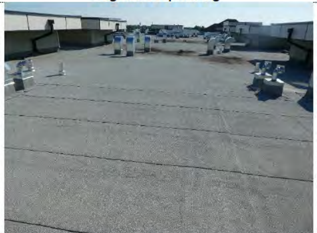
SBS roofing with ridging
