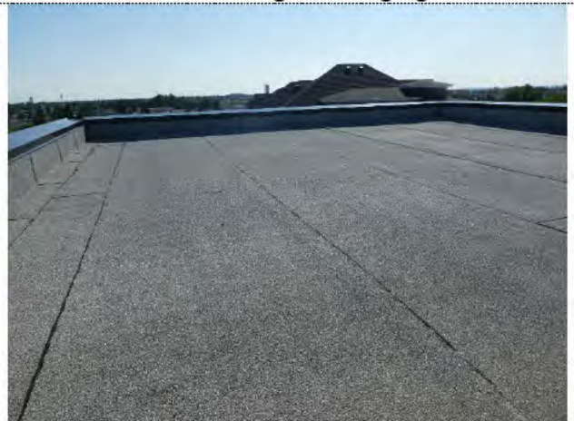
SBS roofing on "loft" section of roof
