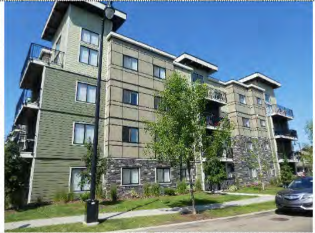
Panel board, siding & stone veneer
