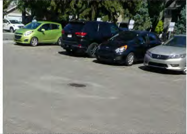
Drain in asphalt
