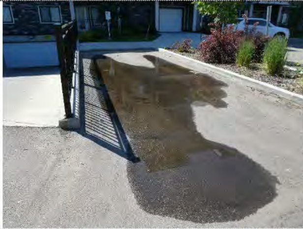
Ponding at garbage truck parking
