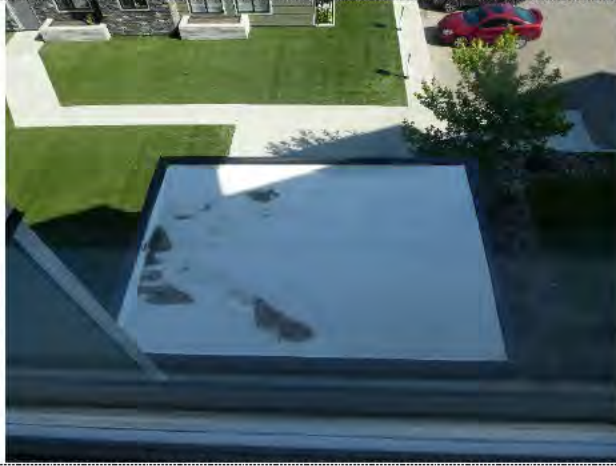
Back entrance canopy roof
