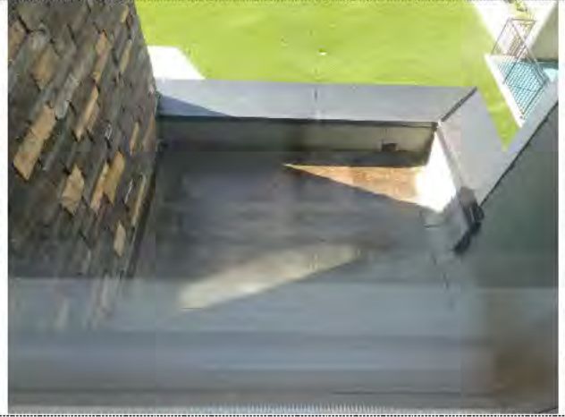
Small roof over stairwell entrance - SBS
