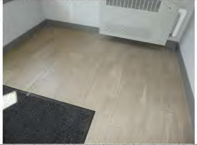
Entrance vestibule tile flooring
