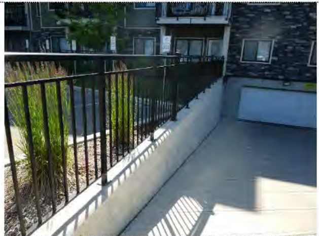
Retaining wall & railings
