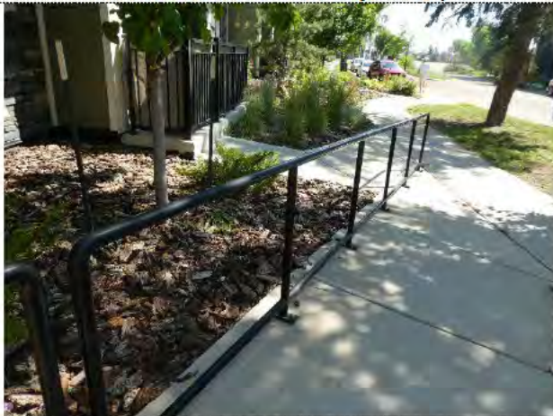
Railings at front of building
