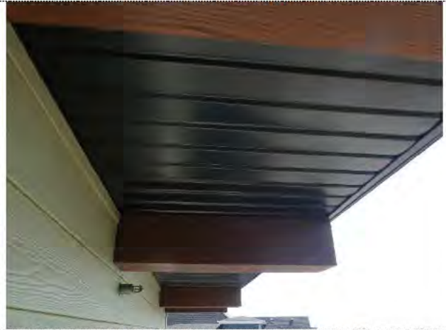
Soffit at loft roof perimeter
