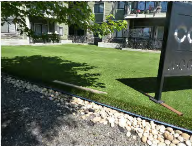
Parkade membrane below artificial grass at SW front of building
