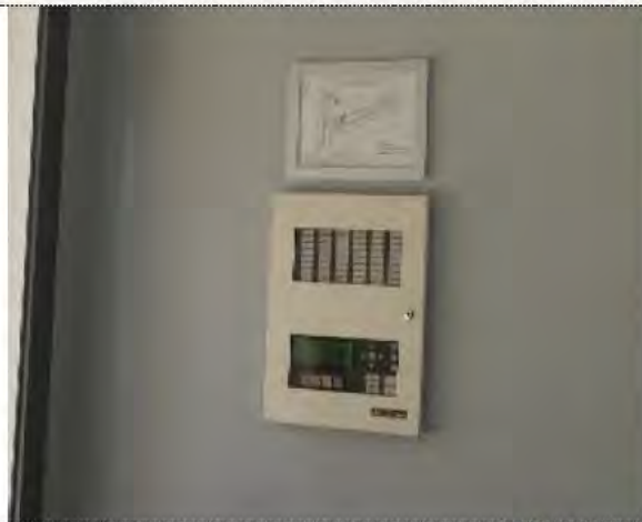
Fire alarm notifier panels
