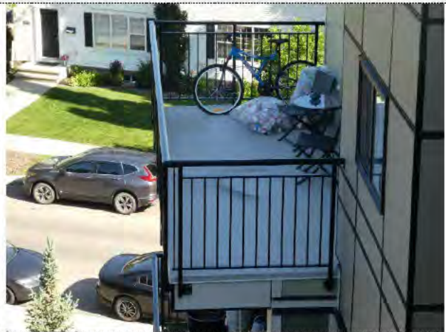
Balcony membrane & railings
