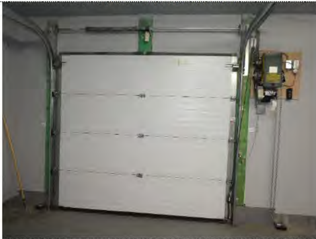
Garbage room overhead door & opener/motor
